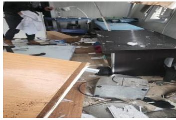
Image: A destroyed treatment room
